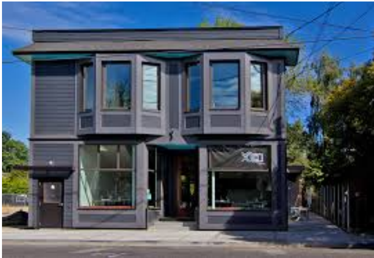
Glasswood Passive House Retrofit, Portland, OR
