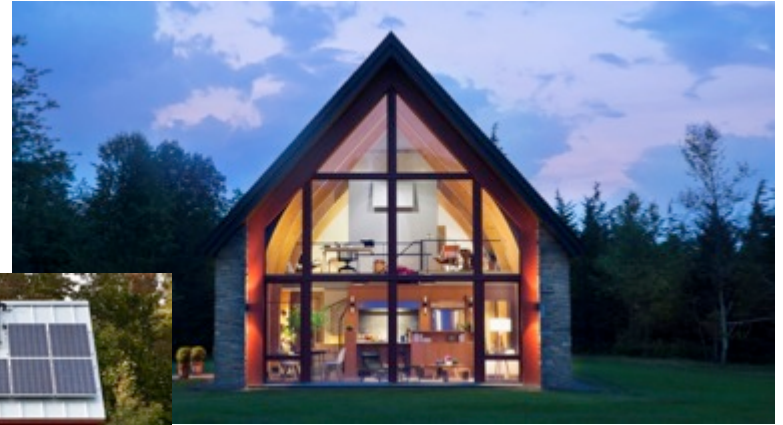
Hudson Passive Project, Hudson, NY
