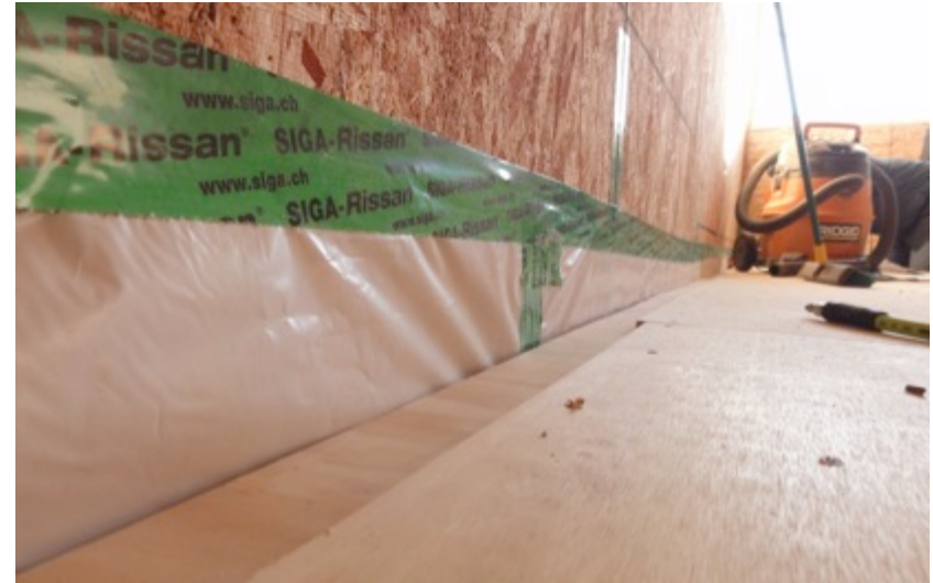
Example of floor to wall connection.
