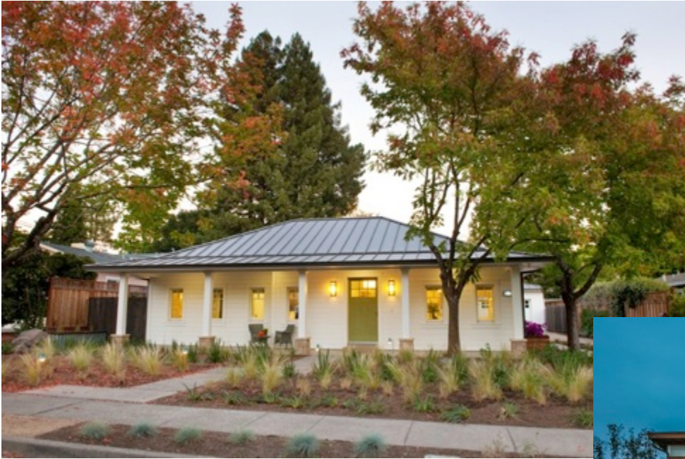
O' Neill House Retrofit, Sonoma, California
