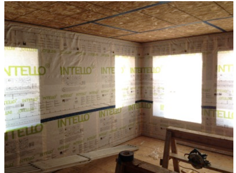
Source: Hayward Design Build
