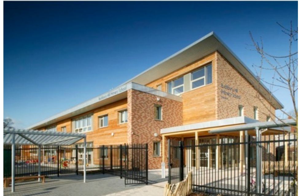
Primary School in the UK (image courtesy: Thomas Vale Construction)
