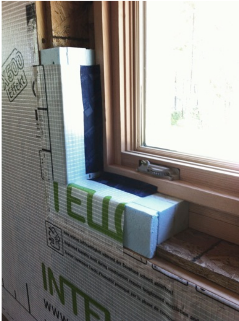
Example of wall to window connection.
